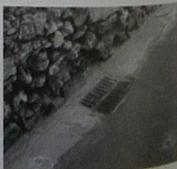
Ravello: Ordinary gutter and drain—just right
